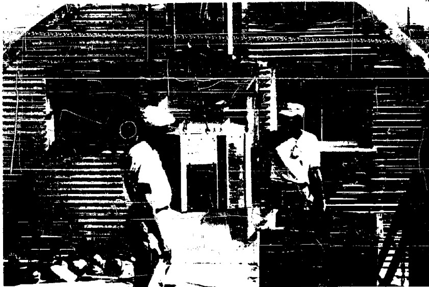
Figure 2.22 Recorder package being transferred from service area to outer magnetic shield box.
